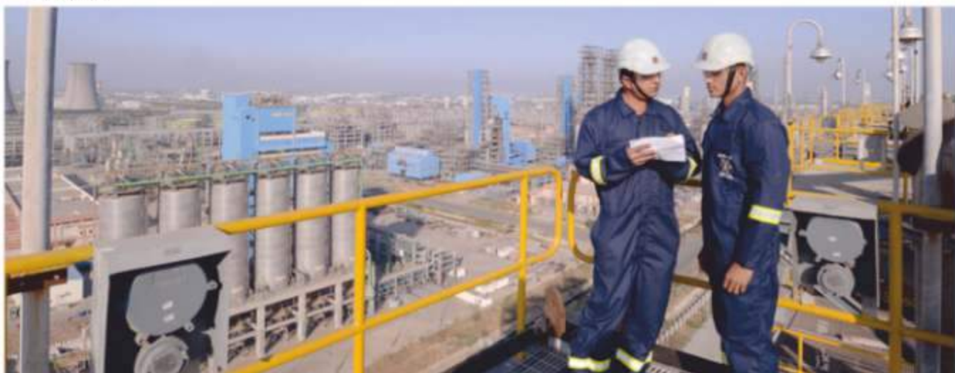
OPaL Plant's view at Dahej
