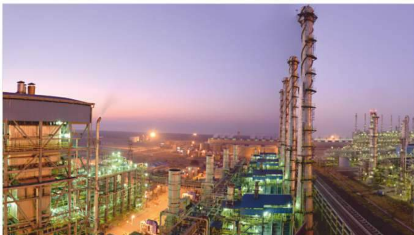
OPaL Plant's view at Dahej
