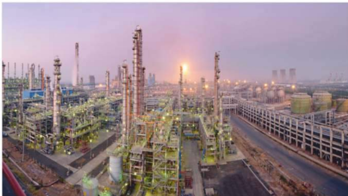
OPaL Plant's view at Dahej
